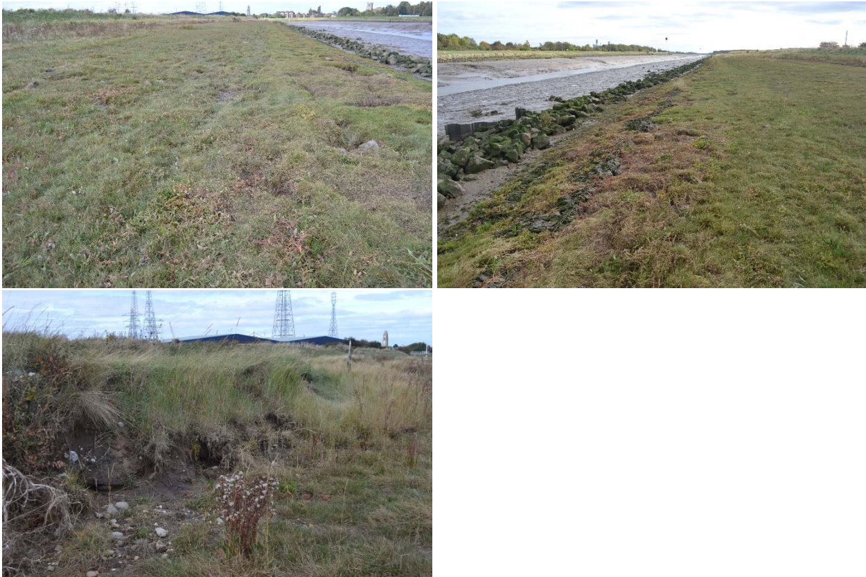
Plate 16.3 Saltmarsh at the Facility (Top) and Exposure of Diamicton at the Facility (Bottom). Saltmarsh Photographs Taken 8 th October 2018 From the West Bank Looking up Estuary (Left) and East Bank Looking Down Estuary (Right).
